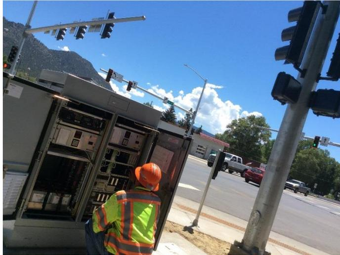
A major component of the project also incorporated the installation of a new traffic signal at the intersection of Main Street and US 24. The new signal includes electronic signalization and detection technology for emergency vehicles. The intersection now also includes enhanced left and right-turn pockets.
